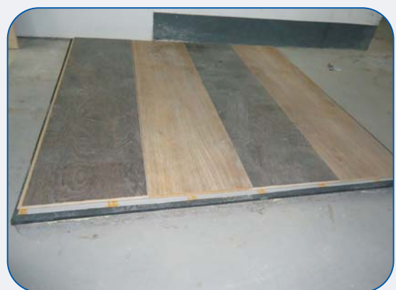
Wood Flooring Installation
