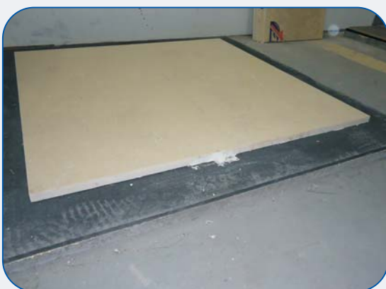
Direct Install under Stone
