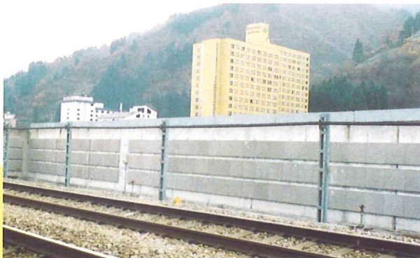
Sound-proof Wall of the New Johetsu Line
